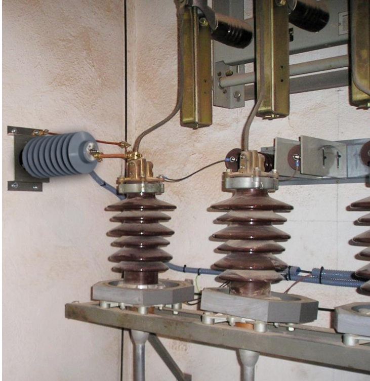
Figure 6 Fastening of a CAMT-5/LS unit using a specific structure in masonry cells
