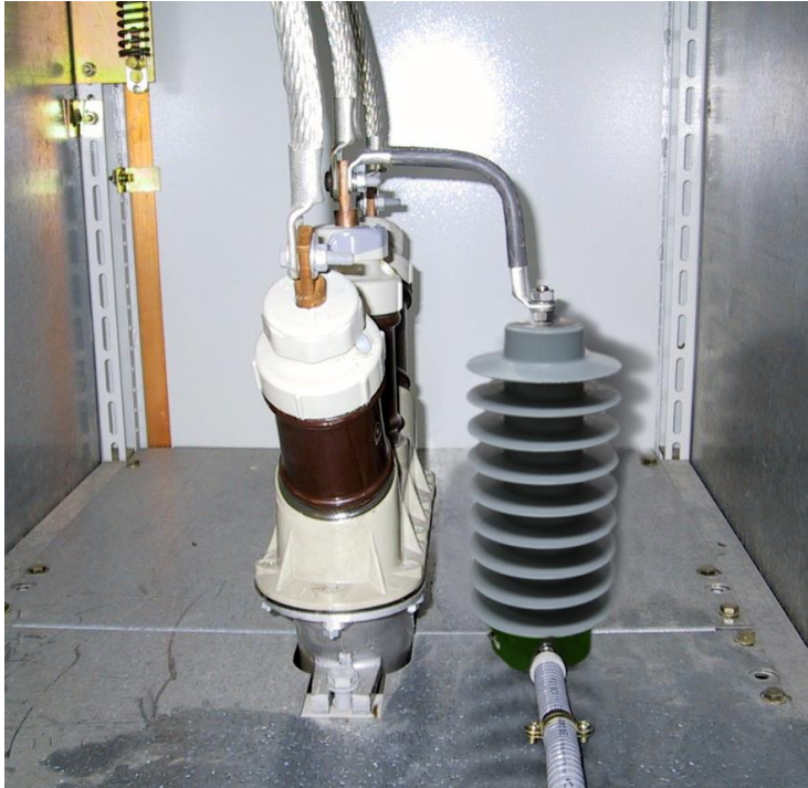
Figure 5 Fastening of a CAMT-5/LS unit using the floor of the cell
