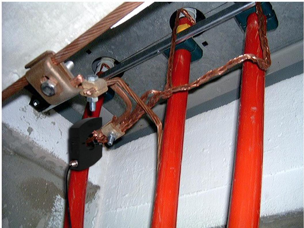
FIGURE 7 Example of installation of the AIBZ-1
