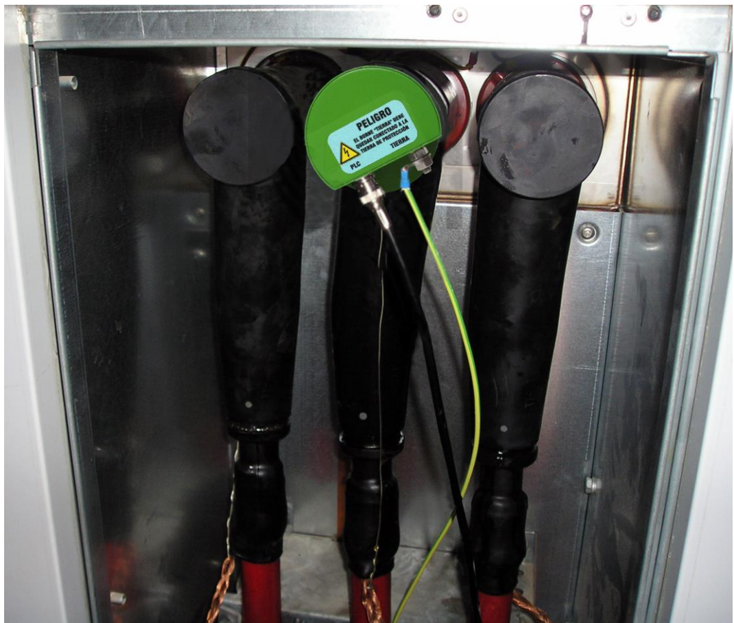
Figure 8 Installation example of the ACA-500 coupler
