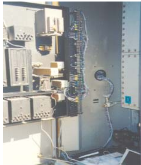
Figure 4: Access Hole and Wiring Harness
